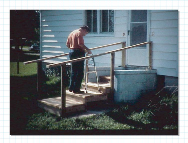
Adding deeper treads to existing steps is beneficial when a person using a walker will us steps. Deep treads are added over existing steps without removing existing treads. This allows easy conversion back to original steps when deep treads are no longer needed.
